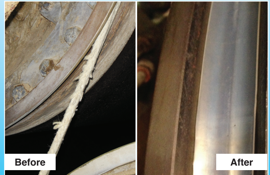
Short rope life remedied by resurfacing rope grooves.
