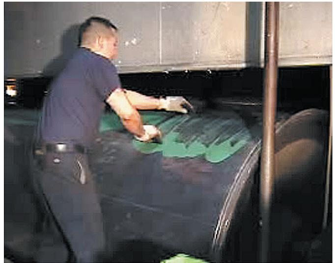
The dryer is then heated up to 250°F (122°C) shrinking down the sleeve.
